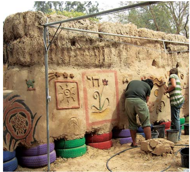
Lotan seminar participants combine environmentally friendly materials such as earth, sand, and fibers to decorate the walls of a children’s workshop space constructed on a recycled car tire foundation.
